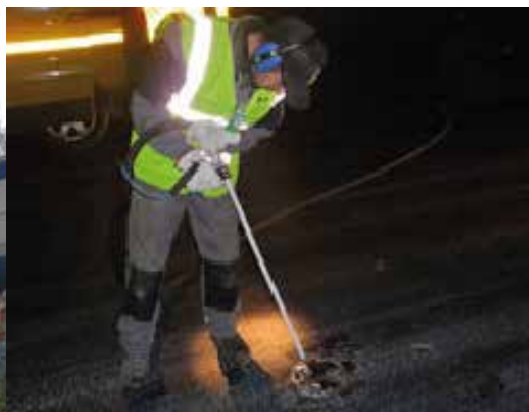
Runway lights cleaning
